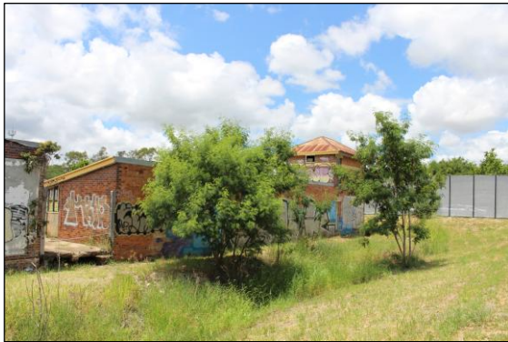
Image 17. West wing west elevation (Jan 26).
