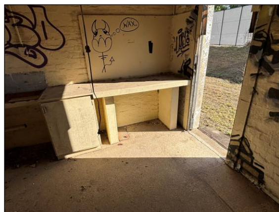
Image 99. Concrete workbench (Apr 26).
