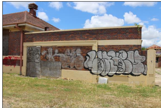
Image 25. North wing north elevation of former waiting shed (Jan 26).
