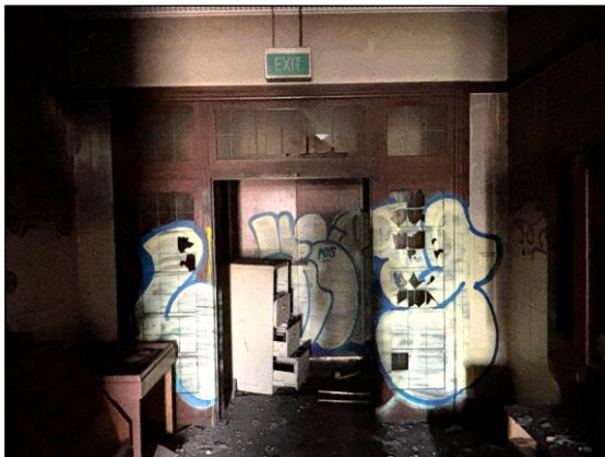
Image 62. East wing entry showing leadlight entry doors with side and top lights (Jan 26).
