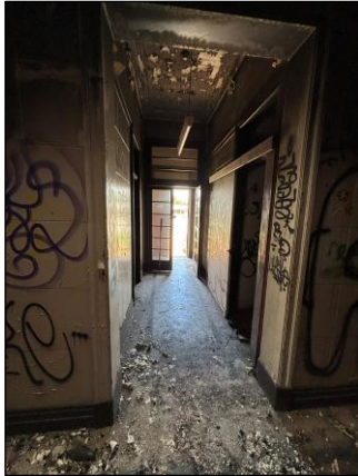
Image 64. East wing entry looking south (Jan 26).
