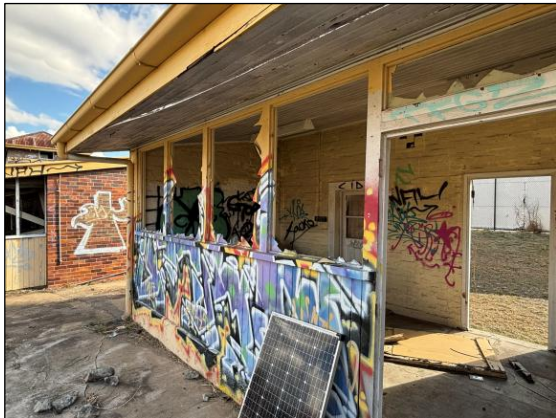
Image 13. North wing east elevation (Apr 26).
