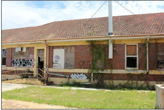
Image 34. North wing part south elevation (Jan 26).
