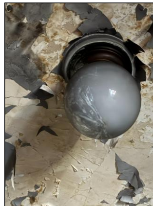
Image 67. East wing entry original light fitting to be salvaged for reuse (Apr 26).
