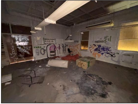
Image 46. North wing operating theatre looking west (Jan 26).
