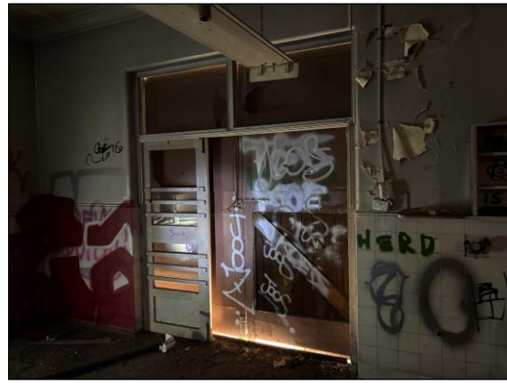
Image 49. Loading doors to western side of operating theatre to external concrete ramp (Apr 26).
