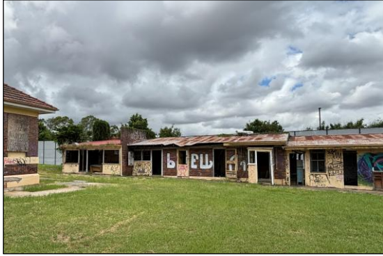
Image 3. South wing north elevation (Jan 26).
