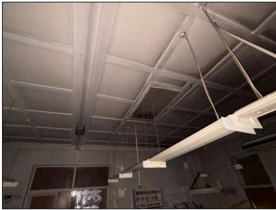
Image 48. North wing operating theatre looking west, typical sheeted and battened ceiling now painted white, with steel ceiling beam and trolley to be retained centre (Jan 26).
