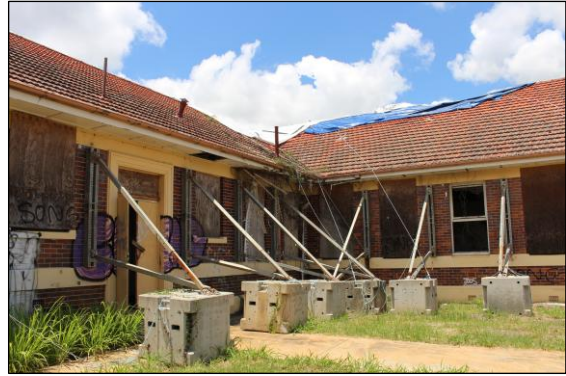
Image 35. Propping to courtyard junction of east and south wings (Jan 26).
