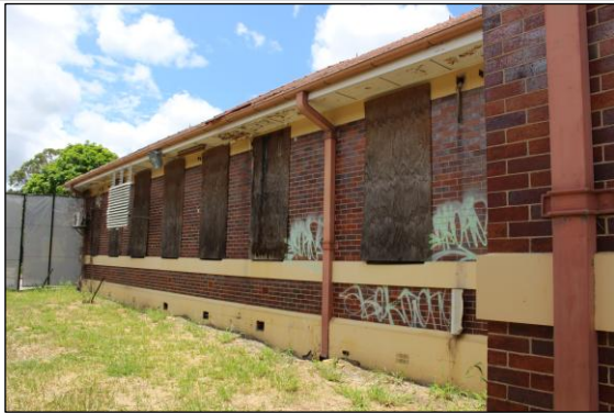
Image 22. North wing part north elevation looking east (Jan 26).
