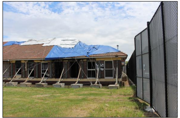
Image 31. South wing part south elevation (Jan 26).
