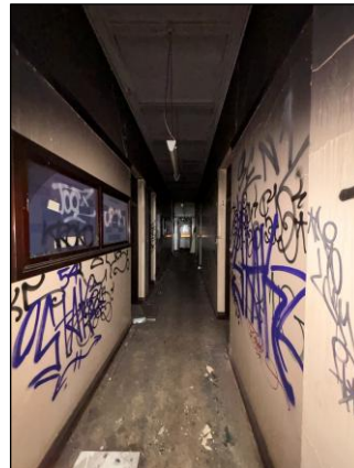
Image 61. East wing central corridor looking north (Jan 26).
