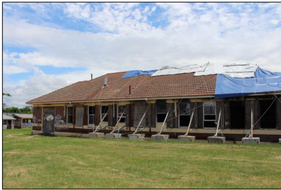
Image 30. South wing part south elevation (Jan 26).
