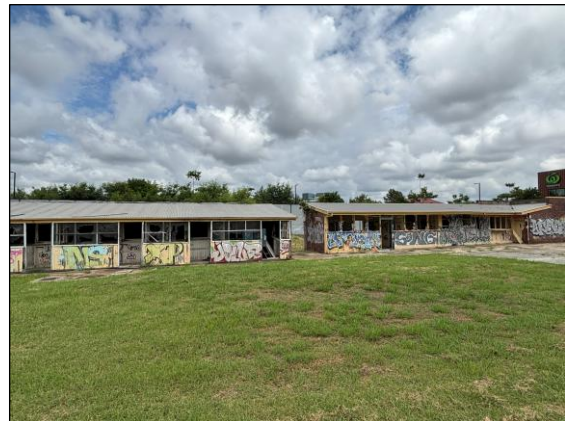
Image 6. West wing part east elevation left and north wing right (Jan 26).
