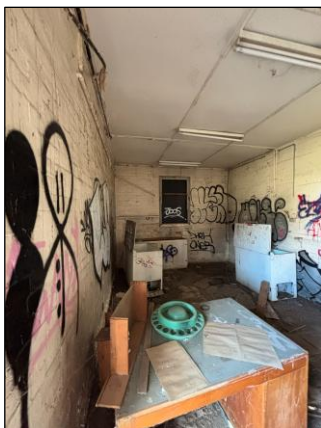
Image 86. Ground floor interior looking south (Apr 26).
