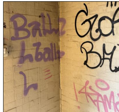
Image 80. Cracks in brickwork (Apr 26).
