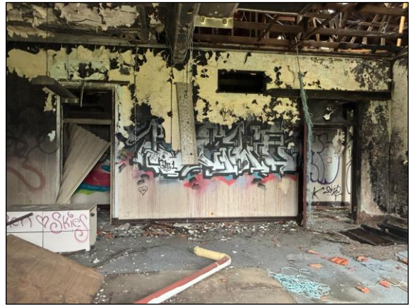
Image 41. South wing fire damage viewed from an external window (Jan 26).
