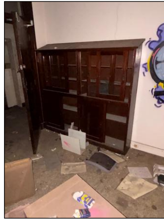
Image 55. North wing example of fixed timber furniture to be retained (Jan 26).
