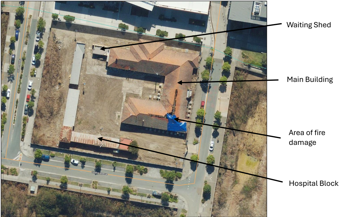
Image ES2. Aerial photograph showing location of fire damage to the roof (Source: Queensland Globe).
