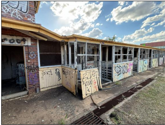
Image 11. West wing east elevation (Apr 26).
