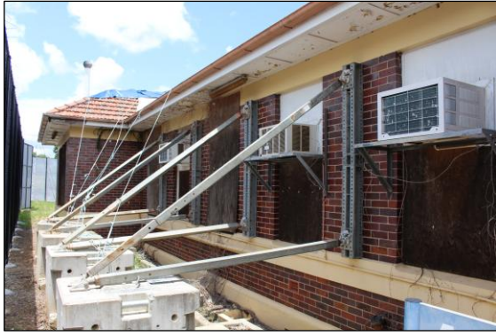
Image 28. East elevation looking south showing propping to southern end (Jan 26).
