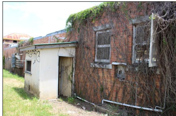
Image 20. South wing south elevation (Jan 26).
