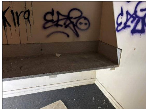
Image 57. East wing, concrete bench to be retained (Apr 26).
