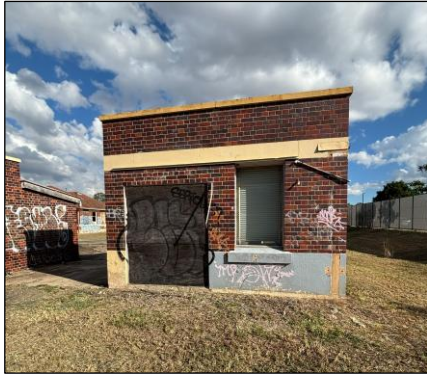
Image 15. North wing north elevation (Apr 26).
