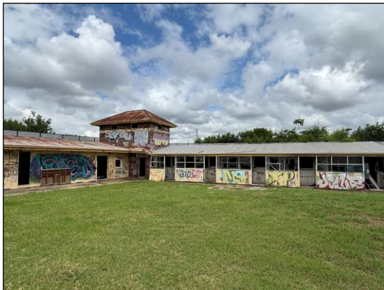
Image 5. West wing part east elevation (Jan 26).
