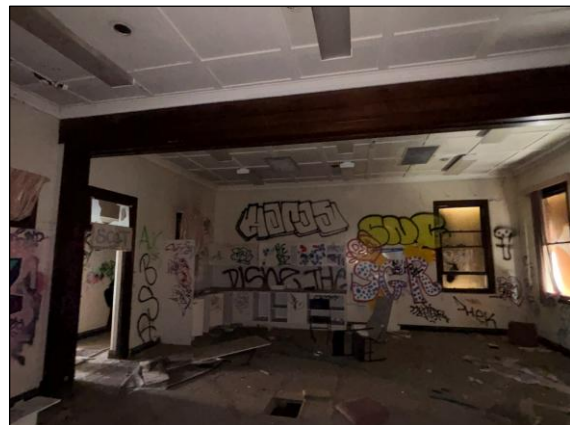
Image 51. North wing meeting room looking west (Jan 26).
