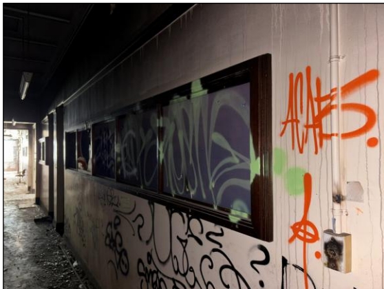
Image 56. East wing central corridor looking south showing noticeboards to be retained (Jan 26).
