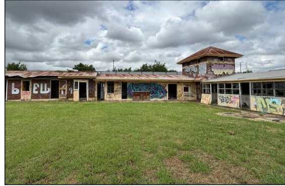
Image 4. South wing north elevation with two-storey fodder store right (Jan 26).
