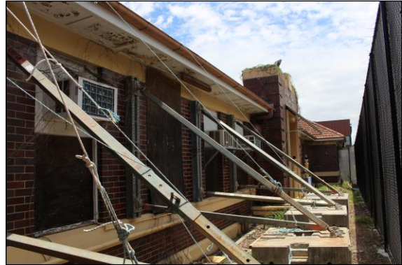
Image 29. East wing east elevation looking north showing existing propping (Jan 26).
