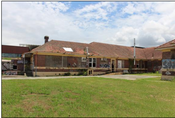
Image 36. North wing south elevation (Jan 26)
