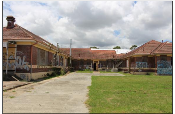
Image 33. Courtyard looking east towards the east wing (Jan 26).
