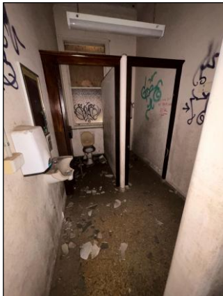
Image 60. East wing toilets with terrazzo flooring, asbestos sheet wall lining and original door frames (Jan 26).
