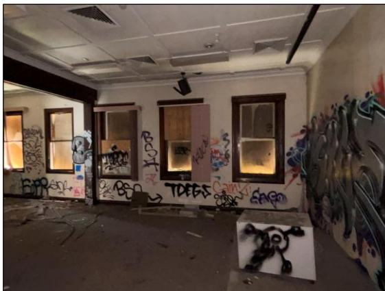
Image 50. North wing meeting room looking north (Jan 26).
