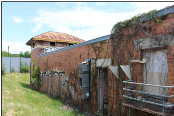
Image 19. South wing south elevation (Jan 26).
