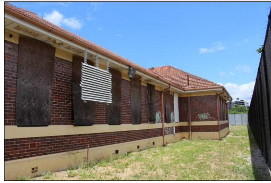
Image 23. North wing part north elevation looking west (Jan 26).
