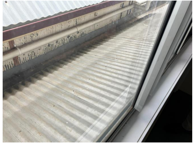
Picture 18 Betty Willis Wing, the roof to the corridor and box gutter to Gowrie House.
