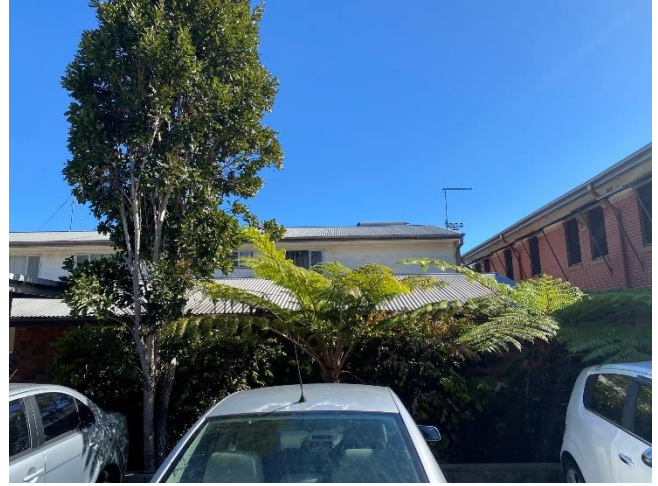
Picture 2 Betty Willis Wing, one and two storey sections, brick and faux weatherboard cladding. The Hoffman-Wadley Wing is to the right.
