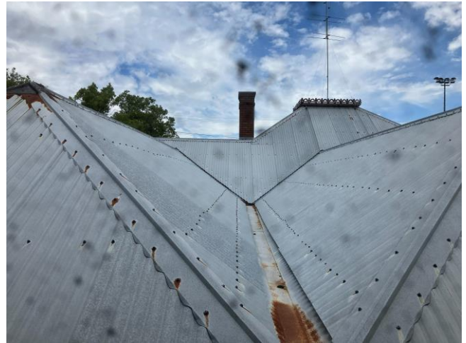
Picture 20 The complex roof form of Gowrie House from the first floor of the Betty Willis Wing.
