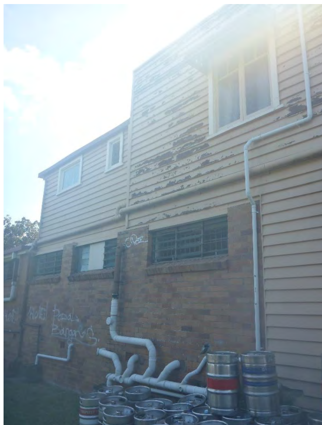
Figure 29: A more detailed view of the circa late-1970s brick addition that was constructed at the northern end of the Clubhouse building during the late 1970s. (Source: VAULT)
