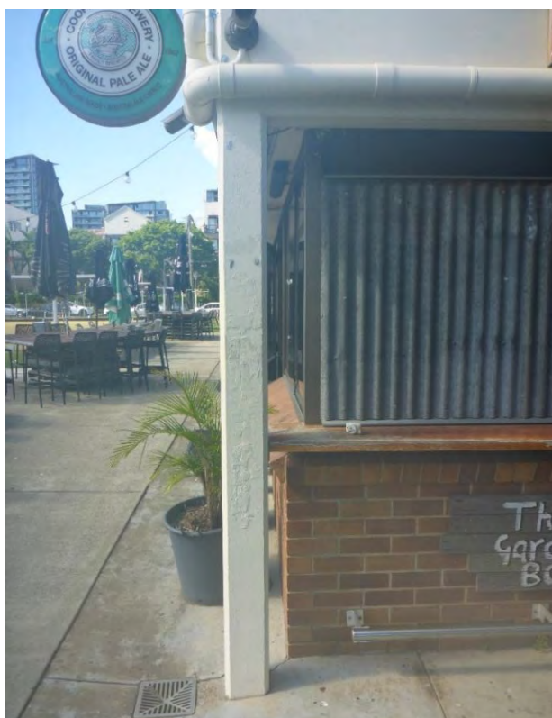
Figure 34: Another detail view of the front (north-eastern) corner of the circa late-1970s forward addition indicating its in-situ concrete frame, face brickwork spandrel panels and aluminium-framed fenestration that infills this concrete frame in order to enclose the ground level within this later addition. (Source: VAULT)
