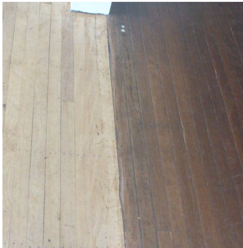
Figure 53: A detailed view of the transition in the timber flooring at the threshold between the original extant of the Clubhouse building – refer to dark coloured timber floorboards at image right – and the timber flooring within the contemporary addition forward of same – refer to light-coloured timber floorboards at image left. (Source: VAULT)
