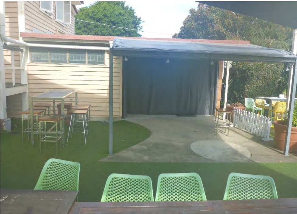
Figure 37: A ground level view of the single storey addition that was constructed at the northern end of the Clubhouse building during the late 1970s / early 1980s. The inboard elevation of this structure is timber weatherboard clad – to match the adjoining Clubhouse exterior - however the balance of the exterior walls are constructed in face brickwork – visible at image far right. (Source: VAULT)
