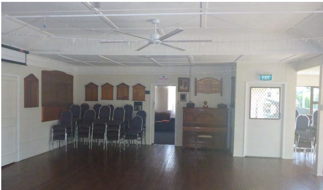
Figure 45: An interior view within the upper level of the Clubhouse building showing the rear / inboard section of that building, which is comprised of the original / early section of this Club facility. The narrow gauge, dark timber floorboards and the batted fibro ceiling of the original building is clearly visible within this interior view. (Source: VAULT)
