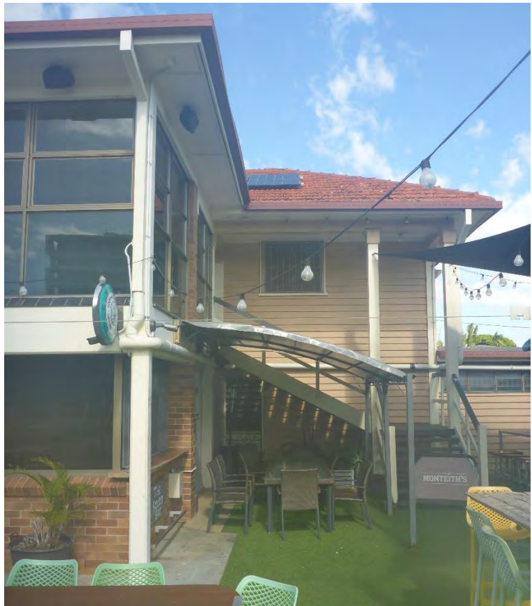
Figure 31: At the north-eastern corner of the Clubhouse building, the transition between the timber weatherboard clad and tile-roofed core of the original Clubhouse building – visible in the background at image centre – and the concrete-framed and fully glazed, double storey extension that is now extant forward of same. (Source: VAULT)
