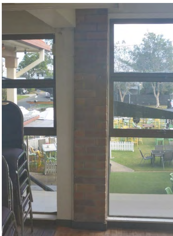
Figure 52: A more detailed view of one of the structural columns extant at the intersection between the original extent of the Clubhouse building – visible at image left – and the contemporary addition made to same during the late-1970s – visible at image right. The doubling up of the structural columns (i.e. original and contemporary) at the transition point between respective phases of development is clearly visible at the centre of this image. (Source: VAULT)
