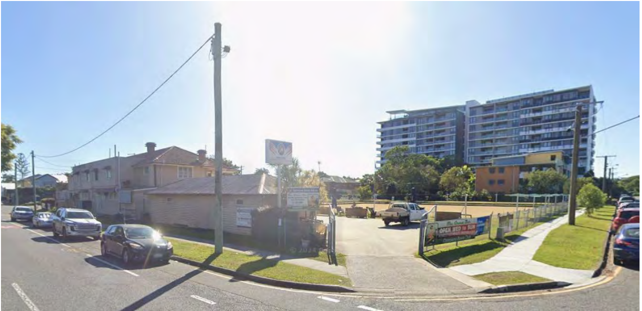
Figure 43: A recent StreetView image – taken in June 2022 – showing the south-western corner of the subject site extant at the intersection of Harries Road (visible at image left) and Wakefield Street (visible at image right). At image centre is the sole vehicular point of entry into the subject site, which comprises a driveway cross-over and an adjoining concrete carpark apron. This vehicular entrance has replaced the other pedestrian arbour structure that previously occupied this street corner in earlier times. (Source: Google Maps)
