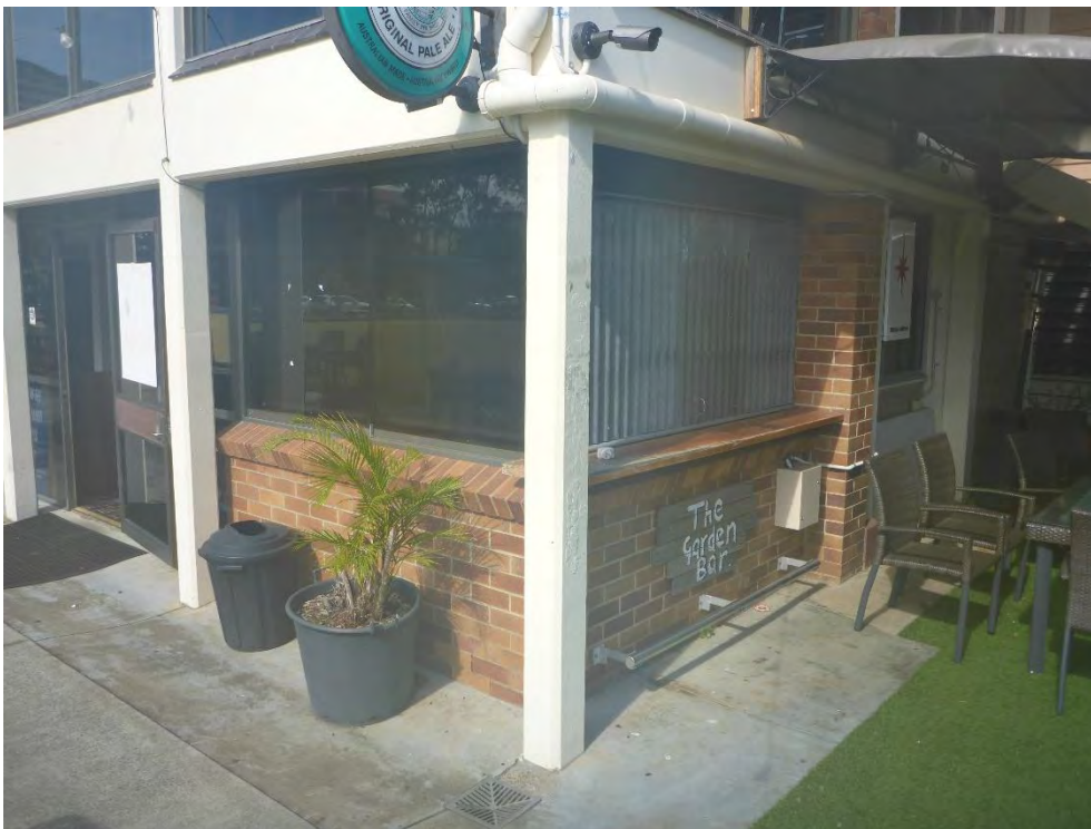
Figure 33: A detail view of the front (north-eastern) corner of the circa late-1970s forward addition indicating the in-situ concrete frame that comprises the “bones” of that later forward addition. This view also indicates the face brickwork spandrel panels and aluminium-framed fenestration that infills the concrete frame in order to enclose the ground level of this later addition. (Source: VAULT)
