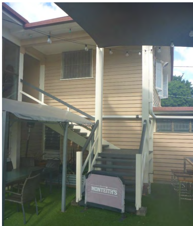
Figure 36: A detailed view of the timber staircase extant at the northern end of the Clubhouse building, which provides access up to the upper level of the Clubhouse and is one of the original / early elements of this building. (Source: VAULT)
