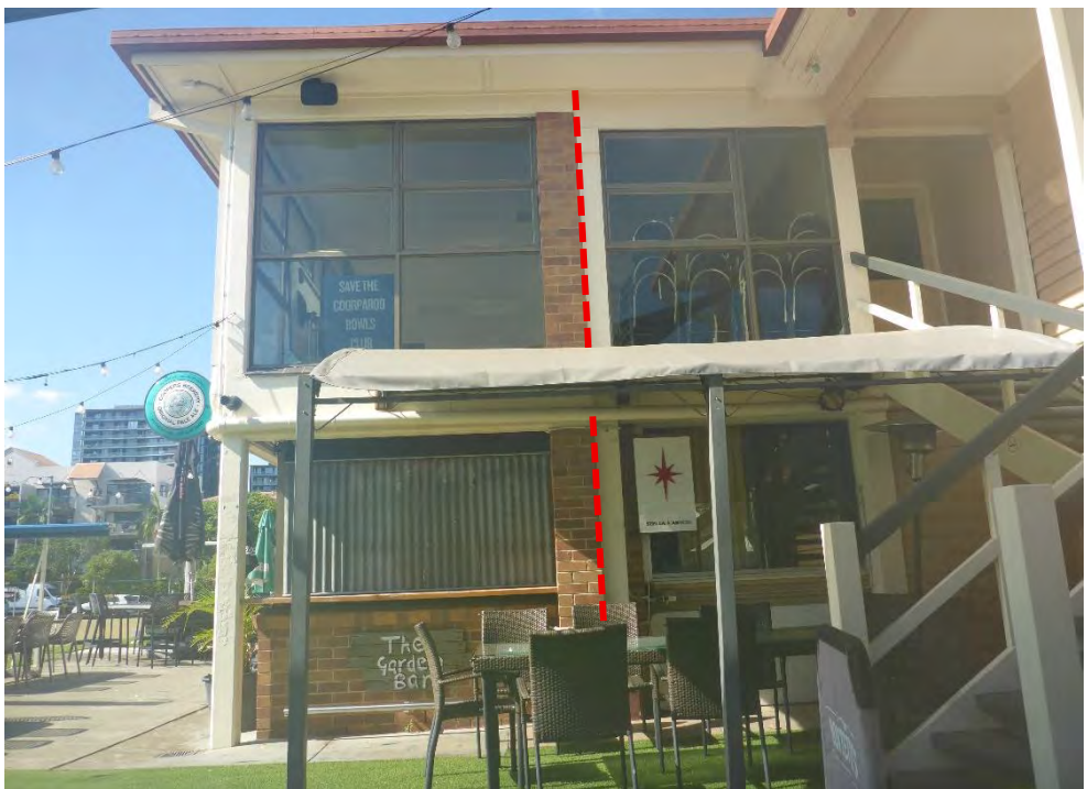
Figure 32: A profile / elevational view of the same north-eastern corner of the Clubhouse building, which serves to illustrate the original extent of this building – visible to the right of the red dotted line – and indicates the forward addition made to same during the late 1970s – visible to the left of the red dotted line. (Source: VAULT)
