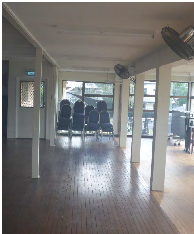
Figure 49: An interior view showing the transition on the upper level of the Clubhouse building between the original extent of this building – visible at image centre and left (with dark-coloured floorboards showing) and the contemporary addition made to same during the late-1970s – visible at image right (with light-coloured floorboards). (Source: VAULT)
