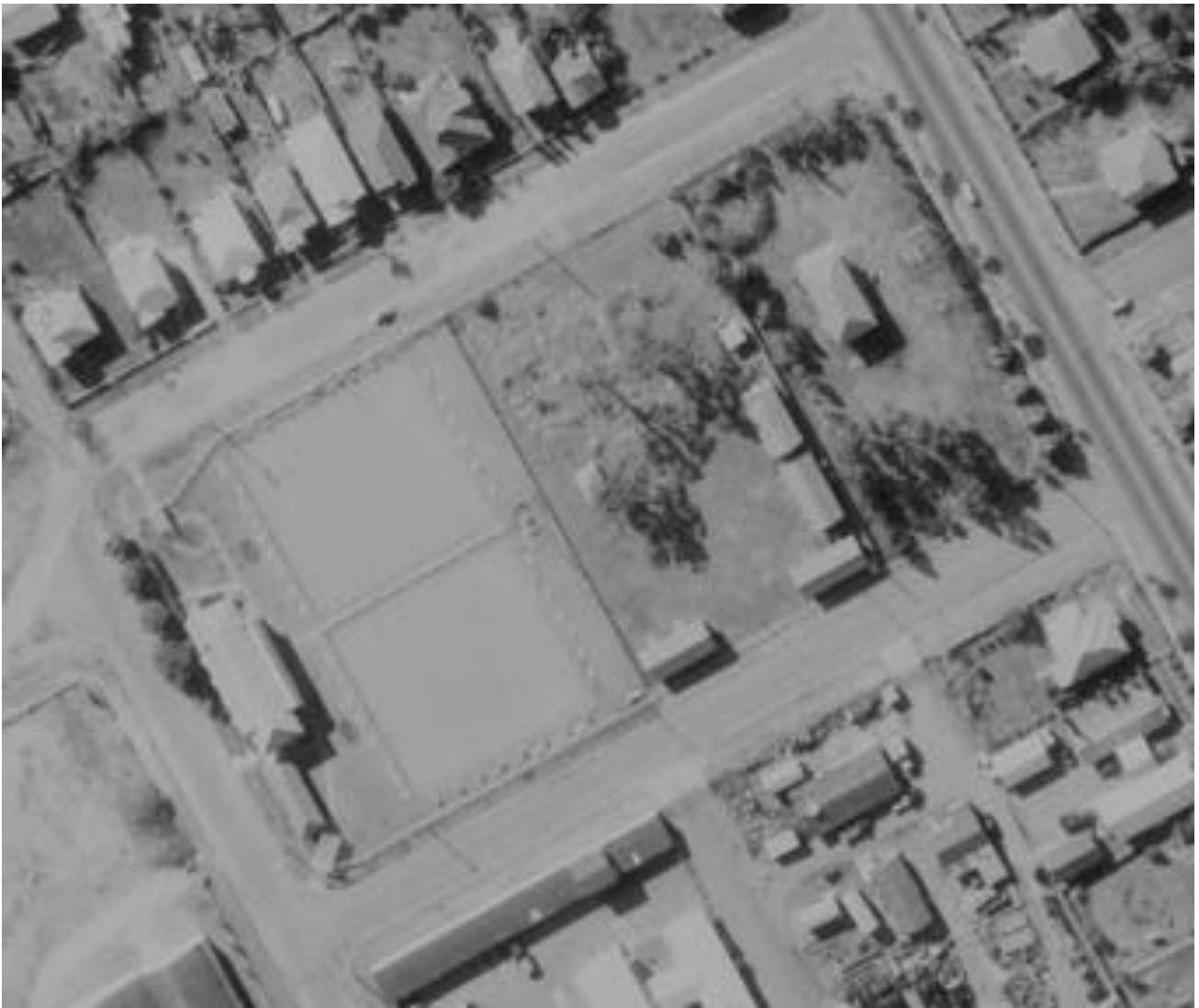
Figure 19: Historical aerial photograph of the Coorparoo area - taken on 16 August 1964 - focussing upon the Coorparoo Bowls Club site and showing the surrounding street grid of Cavendish and Harries Roads, Riddings and Wakefield Streets at its perimeter. (Source: Q Imagery )
