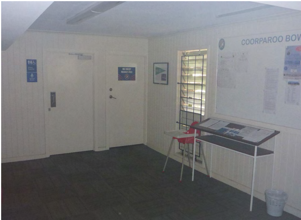
Figure 67: Interior view showing a section of the rear of the ground level of the Clubhouse building, which integrates bathroom and private Club spaces within same. The low ceiling height inherent within this section of the building is once again readily apparent. (Source: VAULT)
