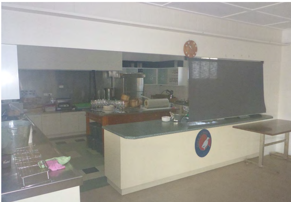
Figure 48: A more detailed view of the commercial kitchen / servery installation extant within the rear / inboard section of that Clubhouse building. (Source: VAULT)
