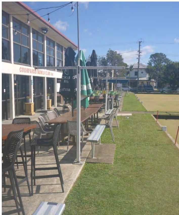
Figure 38: The view looking north across the front edge of the two lawn bowls rinks – shown at image right – and indicating the double storey, concrete framed and fully glazed forward addition that was made to the original Clubhouse during the late 1970s – visible at image far left. (Source: VAULT)
