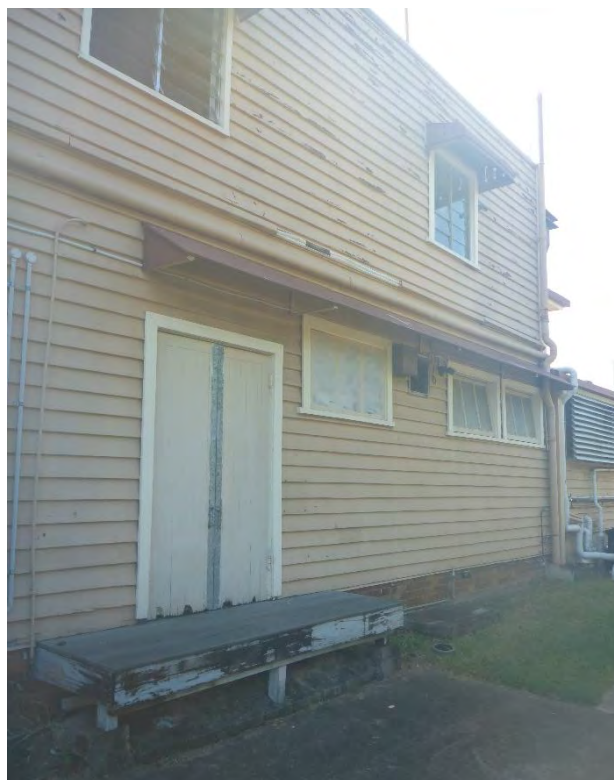
Figure 30: The Harries Road street elevation of the Clubhouse building also incorporates a two-storey, weatherboard-clad exterior wall, which incorporates a small loading dock facility – at image left - within same in order to facilitate the loading / unloading of food and beverage supplies. (Source: VAULT)
