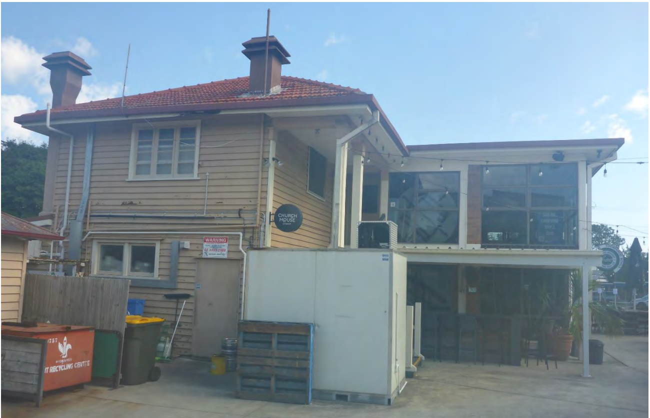
Figure 39: A profile view of the southern end of the Clubhouse building of the Coorparoo Bowls Club site, which clearly indicates the original extent of this building (i.e. timber clad, hipped roof etc. – visible at image left) and contrasts same with the late-1970s forward addition that has significantly expanded the Club’s hospitality offering across both level of the building. (Source: VAULT)
