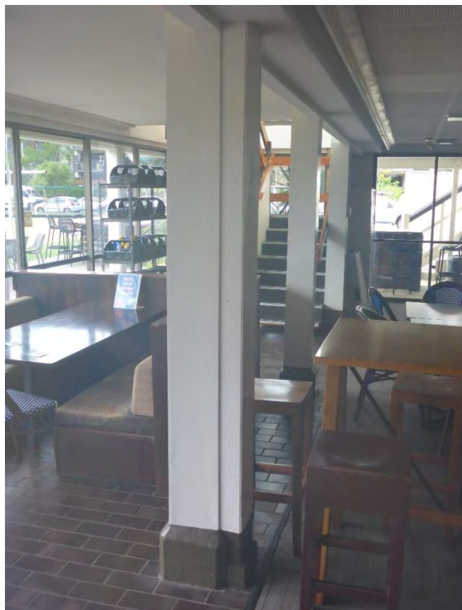
Figure 64: An interior view of the row of concrete columns that align with the original extent of the Coorparoo Bowls Club building and support the upper level of same. The subsequent forward addition and associated enclosure of this ground level space still reveals the original form and detailing of this masonry support structure – visible at the base of the column. (Source: VAULT)
