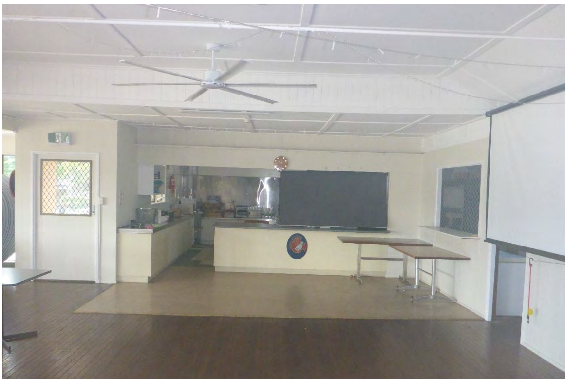
Figure 47: The reverse interior view within the upper level of the Clubhouse building showing the commercial kitchen / servery installation extant within the rear / inboard section of that building. Once again, the narrow gauge, dark timber floorboards and the batted fibro ceiling of the original building is clearly visible within this interior view. (Source: VAULT)
