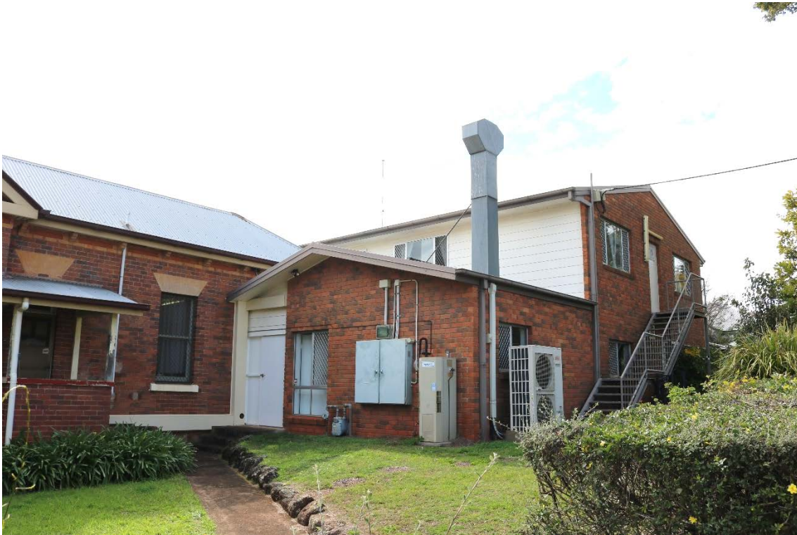
Figure 3: Betty Willis Wing from Arthur Street (Queensland Government, 2026)
