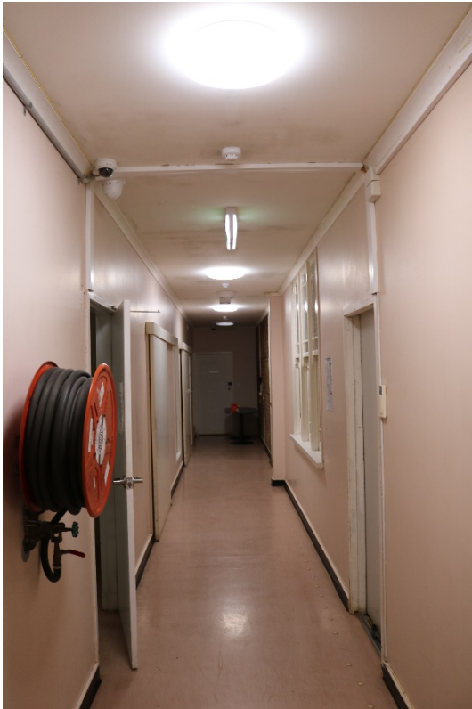
Figure 7: Ground floor, main corridor, looking south (Queensland Government, 2026)
