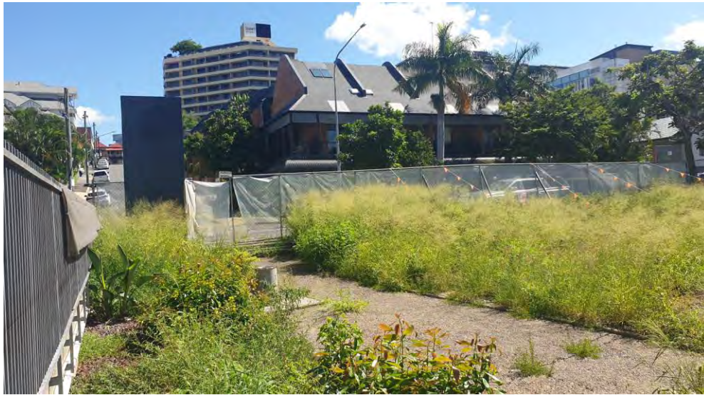
View 30: View of concrete pavement and fence on upper terrace – looking south
