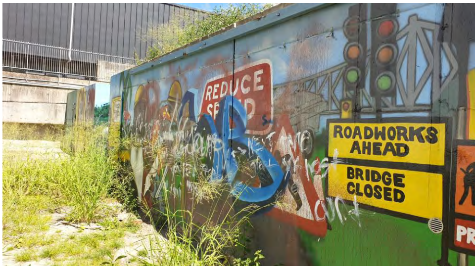
View 11: View of concrete retaining wall on middle terrace – looking southeast
