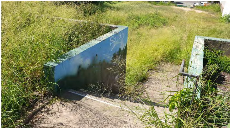
View 24: View of concrete pavement and stair in upper terrace – looking north
