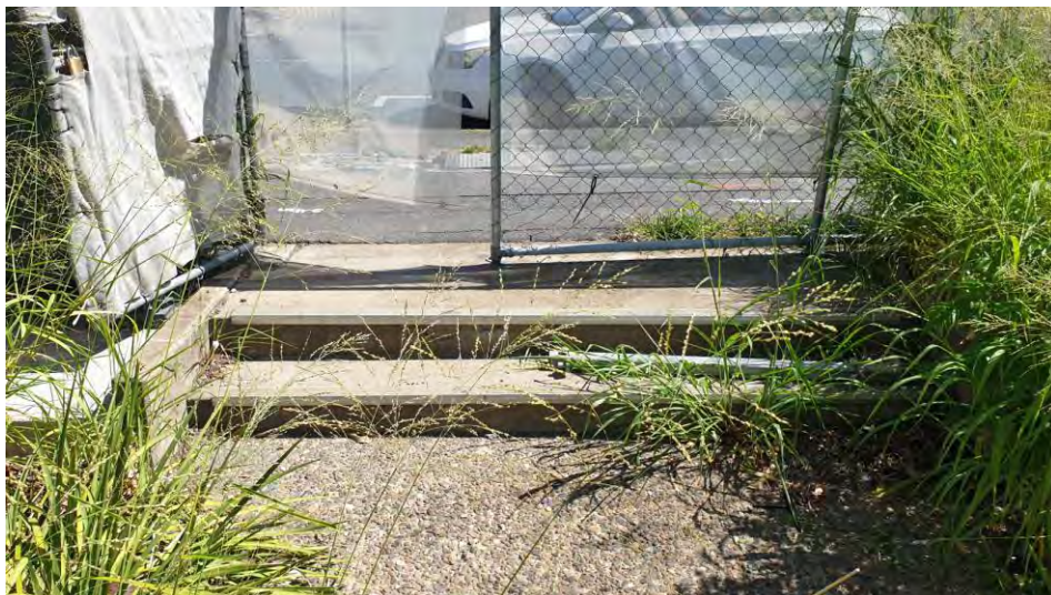
View 26: Concrete steps connecting upper terrace to footpath along Boundary Street
