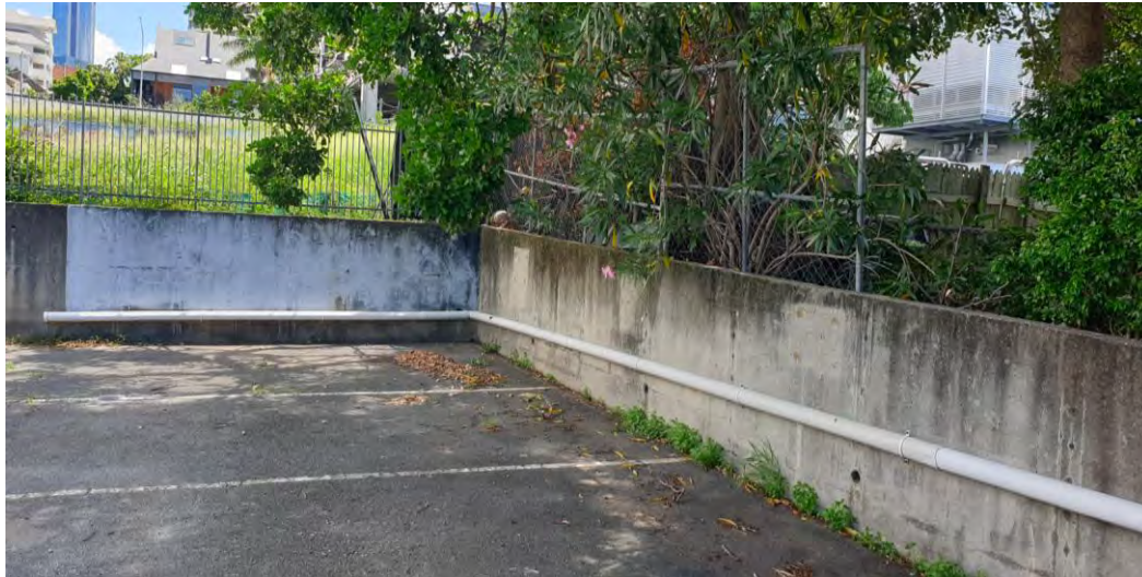
View 2: Concrete retaining wall and boundary wall on lower terrace (car park)
