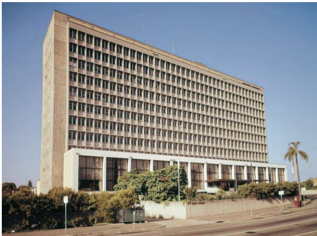
Figure 10: Main Roads Department Head Office complex, c. 1970s (Source: TMR)
