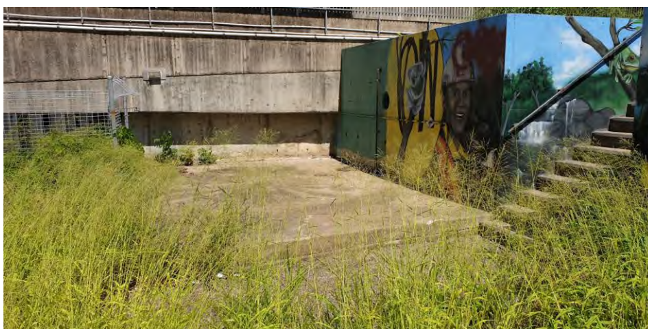
View 12: View of concrete pavement, retaining wall and stair on middle terrace – looking southeast
