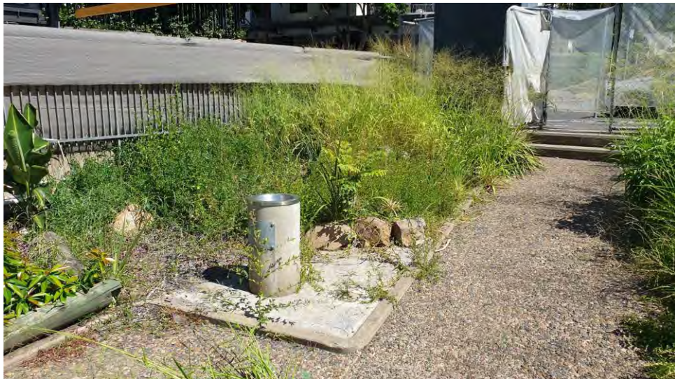
View 25: View of concrete pavement and drinking fountain in upper terrace – looking south
