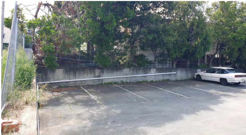
View 5: Concrete retaining wall and boundary wall on lower terrace (car park) – looking northwest
