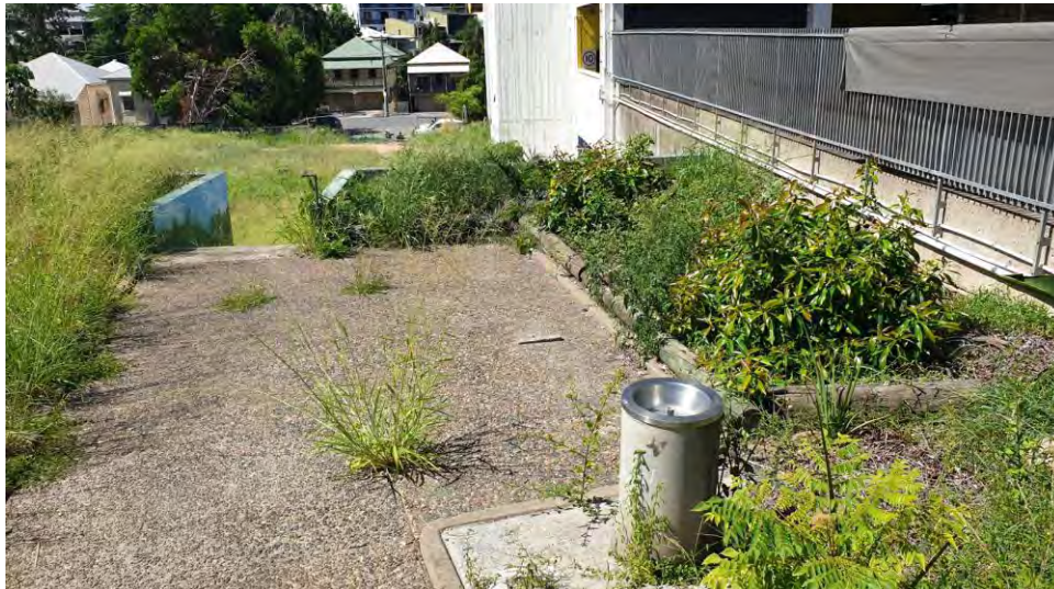
View 22: View of concrete pavement and drinking fountain in upper terrace – looking north
