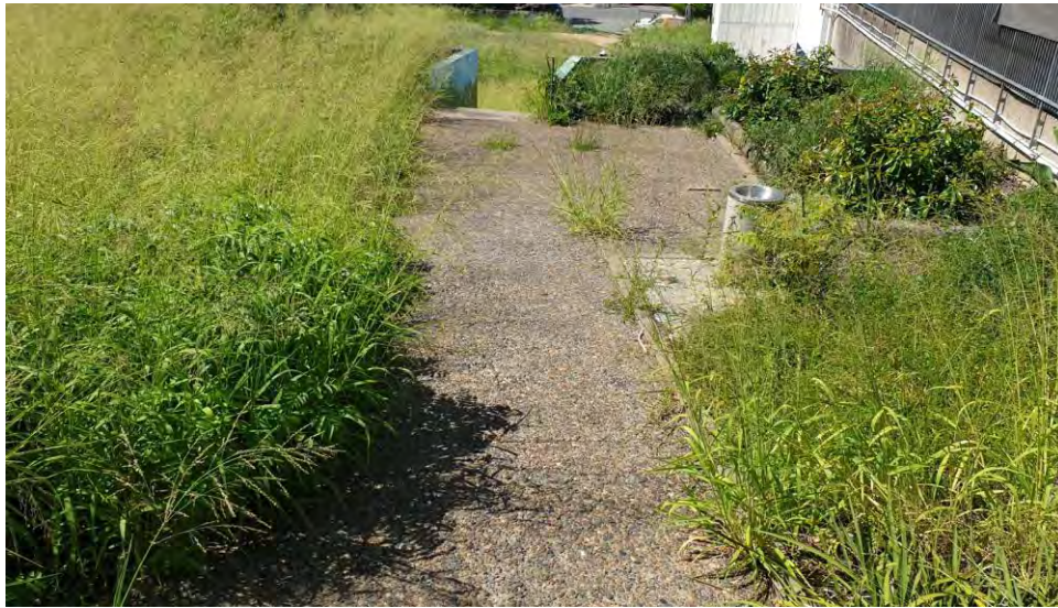
View 21: View of concrete pavement in upper terrace – looking north
