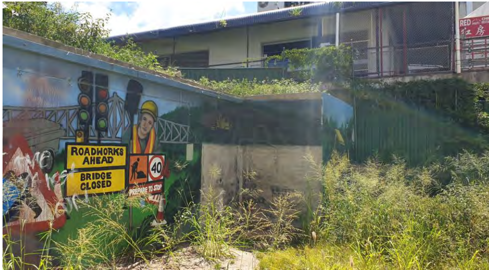
View 10: View of concrete retaining wall on middle terrace – looking southwest
