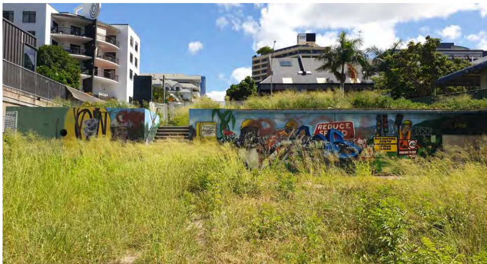
View 9: View of concrete retaining wall on middle terrace – looking south
