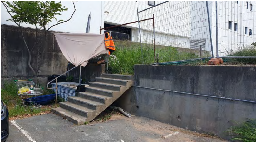
View 4: Concrete retaining wall, stair and boundary wall on lower terrace (car park)
