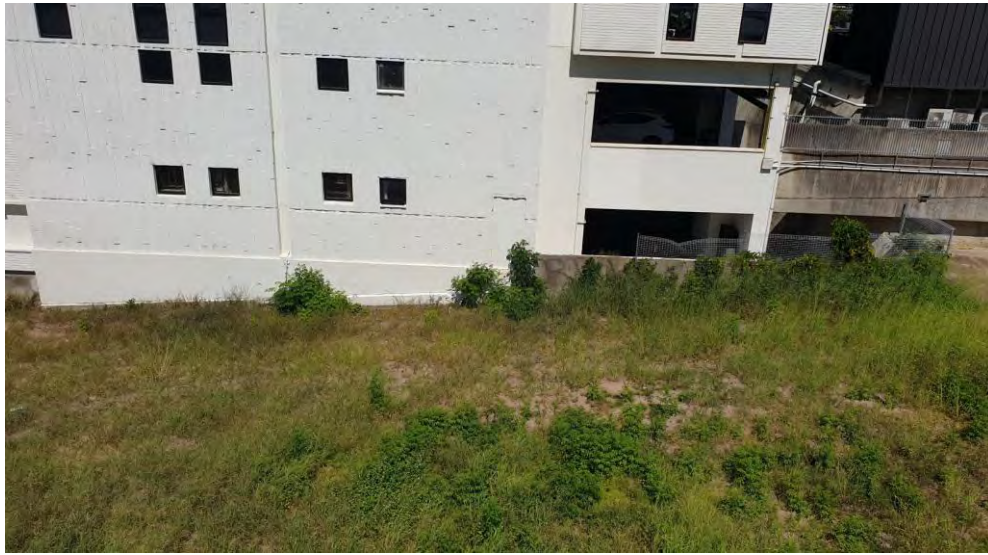
View 18: View of middle terrace – looking east
