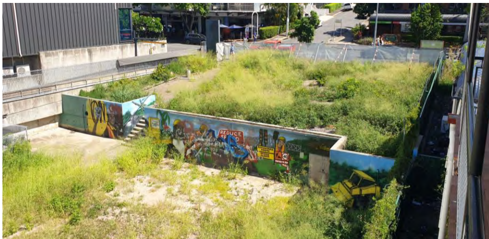
View 17: View of upper terrace and concrete retaining wall – looking southeast
