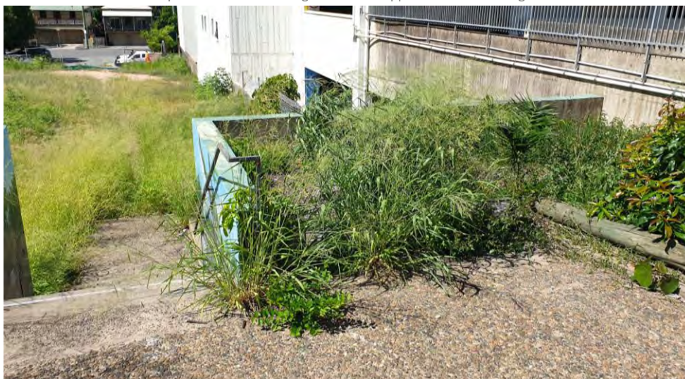
View 23: View of concrete pavement and stair in upper terrace – looking north
