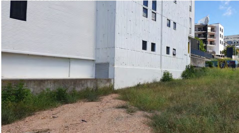
View 8: View of middle terrace – looking southeast
