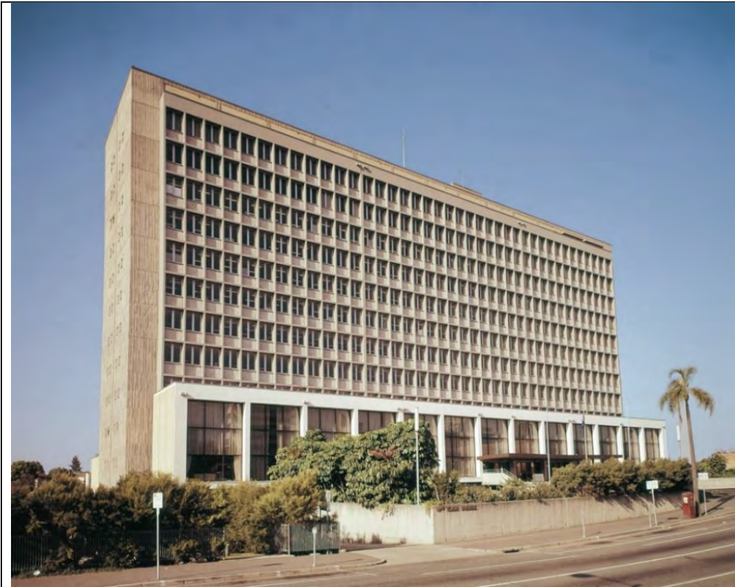
Main Roads Department Head Office complex, c1970s.
