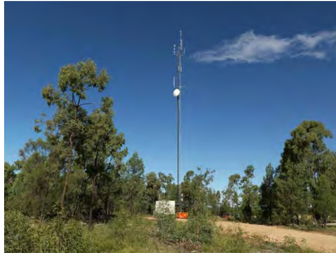
Figure 1-6 Existing communication tower at Talinga
