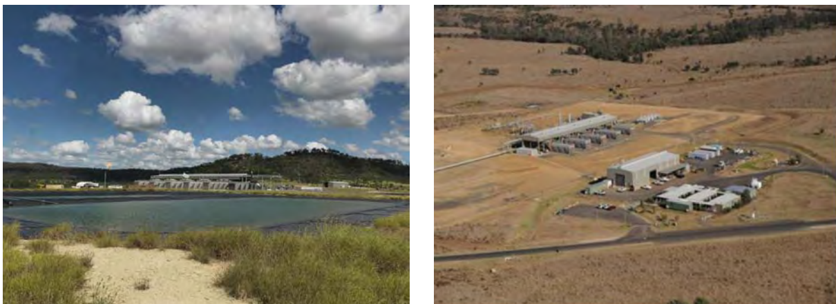
Figure 1-3 Australia Pacific LNG's existing Strathblane and Spring Gully gas plants
