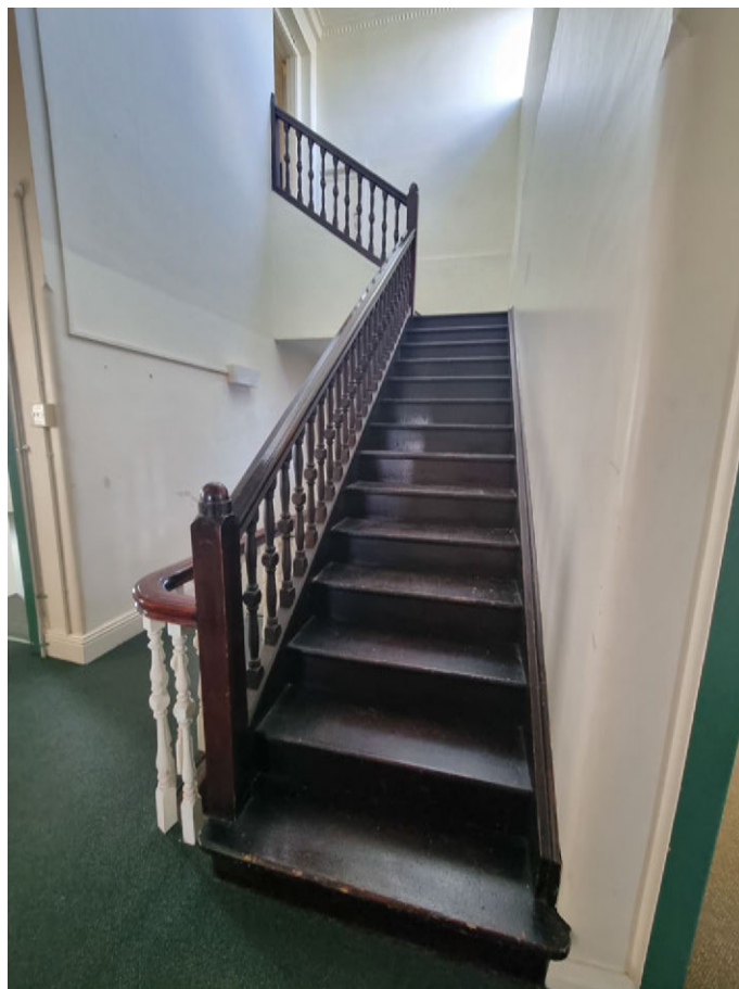
Figure 14: Stair up to second-floor Tower Room (Queensland Government, 2026)
