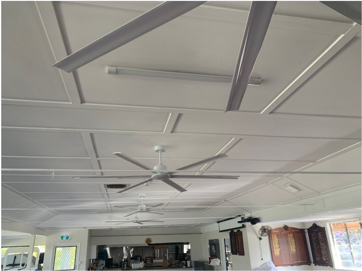
Upper level vaulted plywood panel ceiling with exposed steel tie rods.
