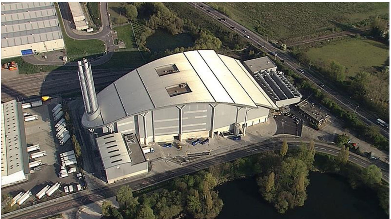
Lakeside facility aerial view. Image available at: https://www.viridor.co.uk/siteassets/images/erf/lakeside-efw/lakeside02.jpg
