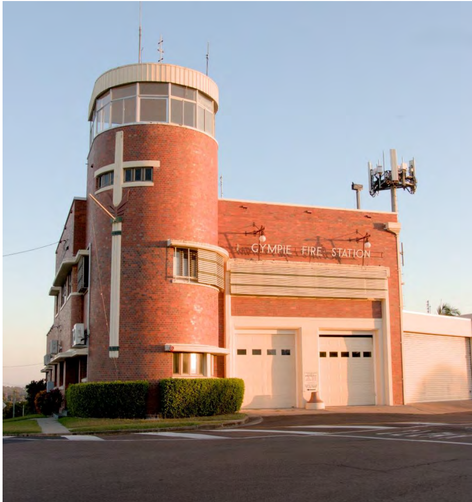
Figure 21 IMG_010 - Gympie Fire Station main building taken from Bligh Street
