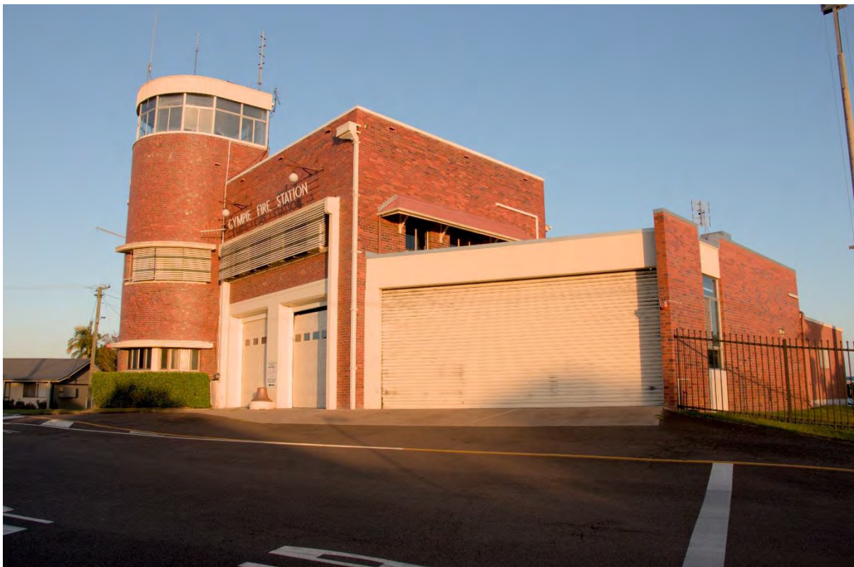
Figure 13 IMG_002 - Gympie Fire Station main building and 1970s additions from Bligh Street showing Bligh Street frontage.
