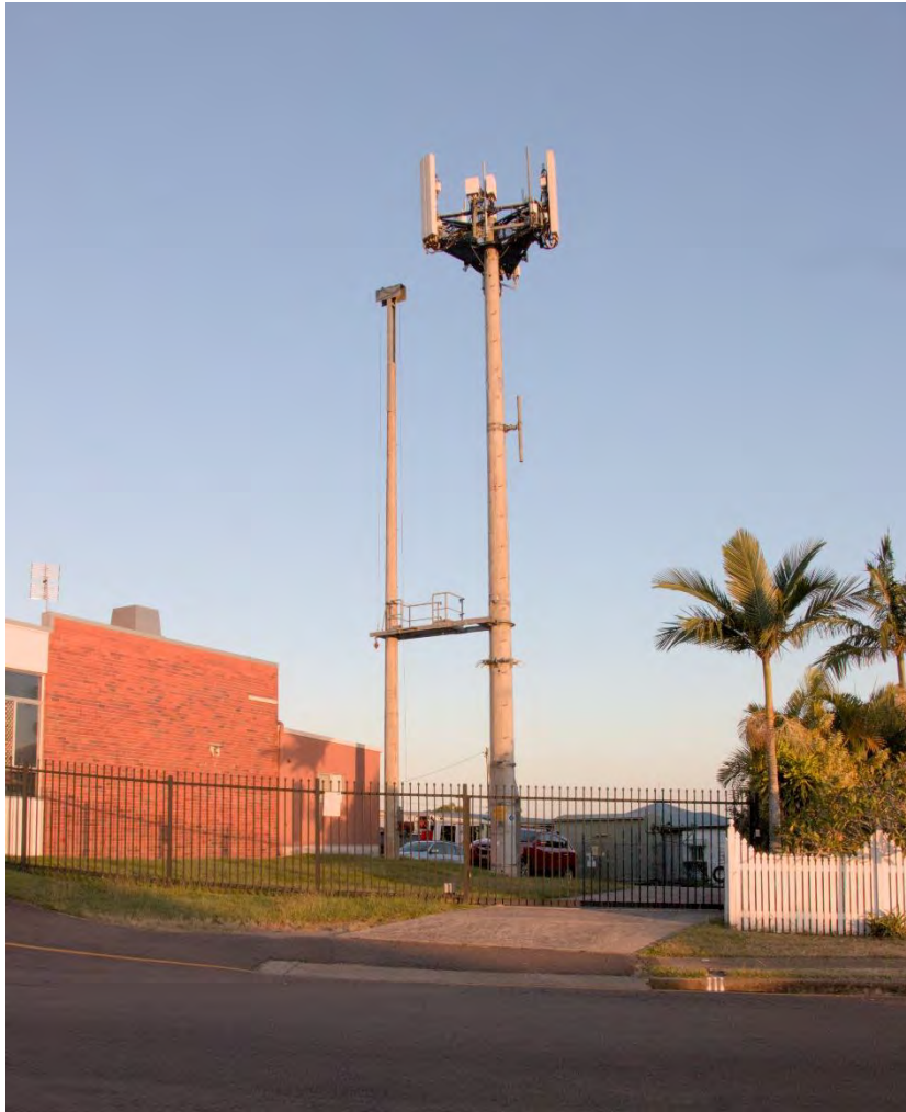
Figure 18 IMG_007 - Communications tower, fencing and BA room taken from Bligh Street.
