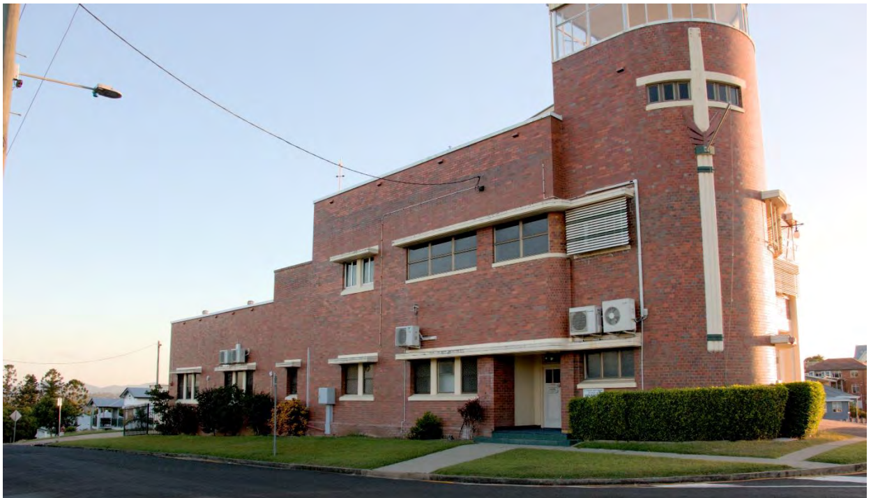
Figure 15 IMG_004 - Gympie Fire Station main building taken from Nelson Road showing Nelson Road frontage.
