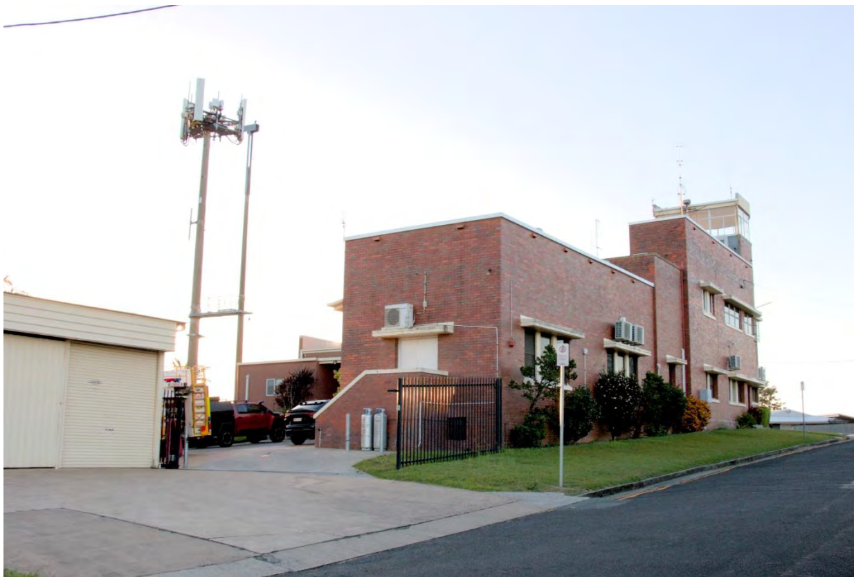
Figure 16 IMG_005 - 005 IMG_005 Rear of Gympie Fire Station main building taken from Nelson Road.
