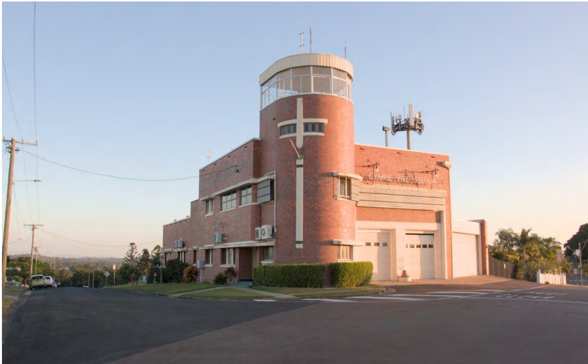
Figure 12 IMG_001 - Gympie Fire Station main building from Bligh Street showing Bligh Street and Nelson Road frontage
