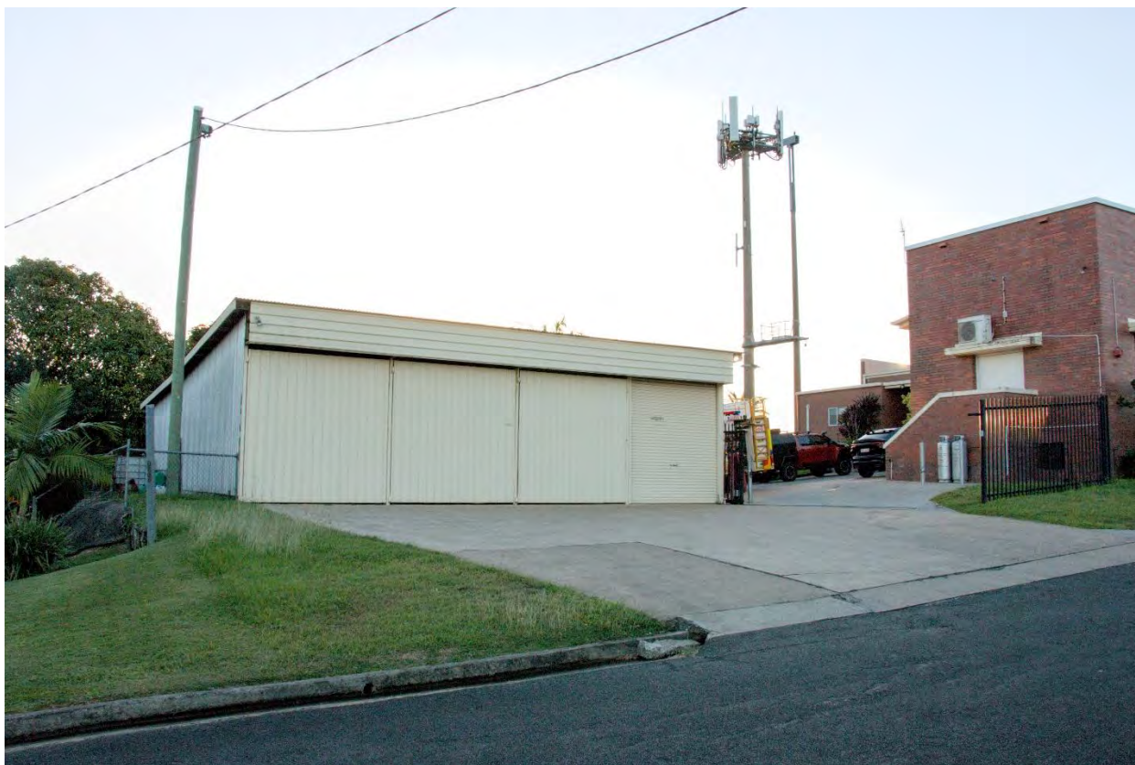
Figure 17 IMG_006 - Gympie Fire Station storage shed and communications tower taken from Nelson Road.
