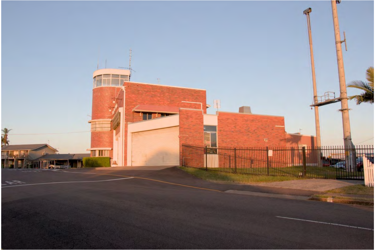
Figure 14 IMG_003 - Gympie Fire Station main building and 1970s additions from Bligh Street showing Bligh Street frontage.
