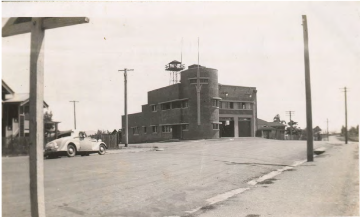
Figure 10 Gympie Regional Library, Gympie Fire Station showing timber tower, pre-1948.
