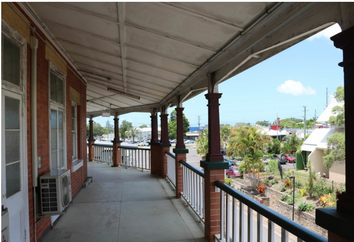
Figure 4: First floor verandah, 1943 wing (Queensland Government, 2024)
