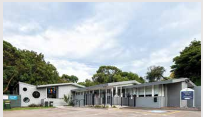
The Montague Park Pre-School & Maternal Welfare Centre was recognised for its post-war heritage significance.
