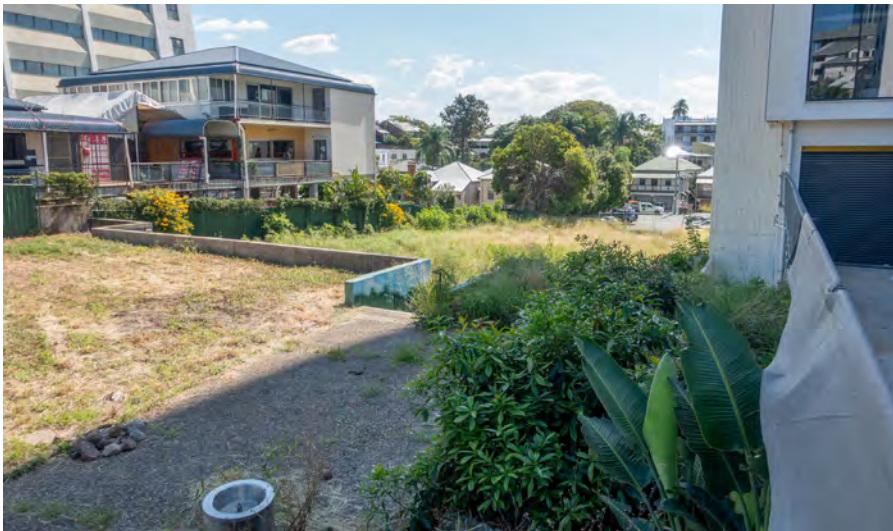
5 Original concrete path at upper level as shown in the original drawing.
