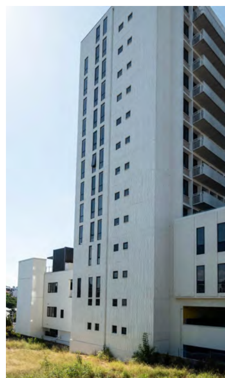
1 Western elevation, former Main Roads Department Building. The open space adjacent was critical to less the impact on the adjacent houses
