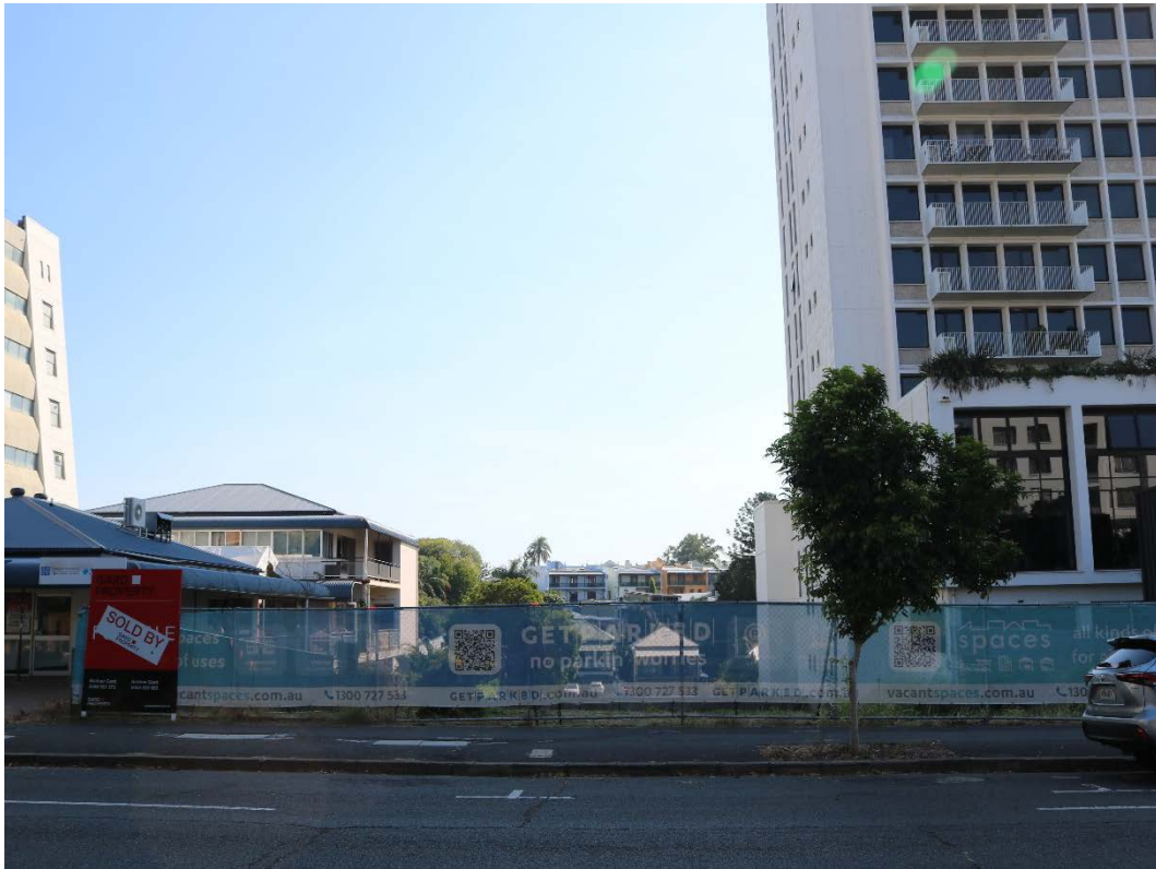
Figure 3: Western garden looking north from Boundary Street with Main Roads Department Building at right (Queensland Government, 2026)
