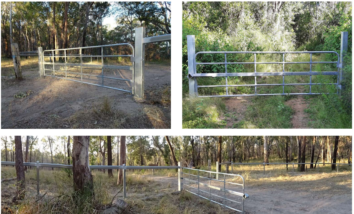
Figure 15: Gates and fencing installed on de-gazetted roads to restrict public vehicle access to Oakview NP. Side barriers have since been installed on the gate in the top right.
