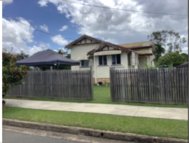
11 Cullen Street – subject property – traditional house to be retained
